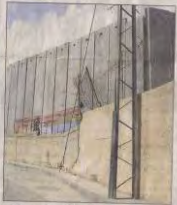
Part of the wall built to protect Bethlehem.
